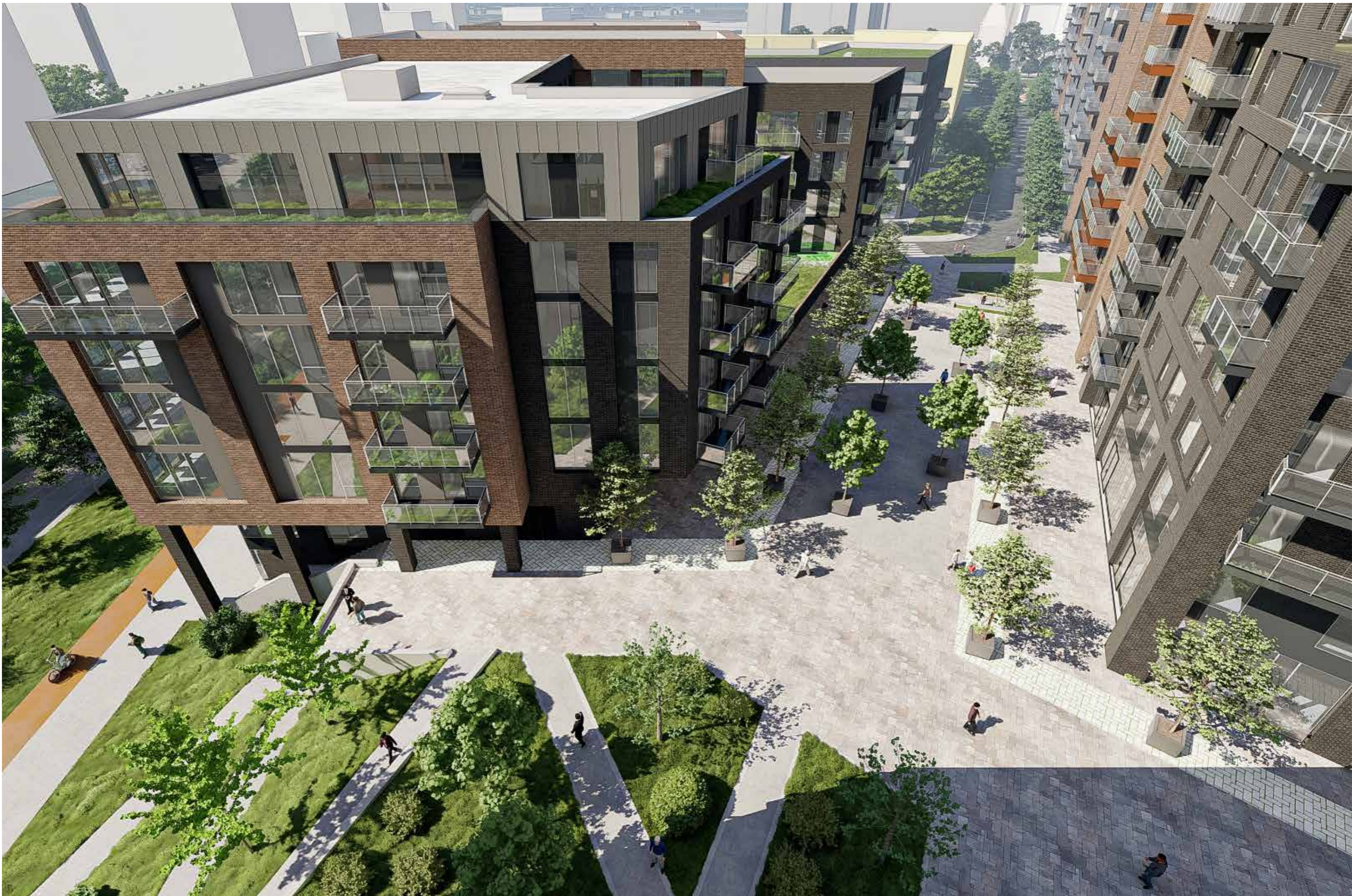
View along Centre Park Road towards tower
