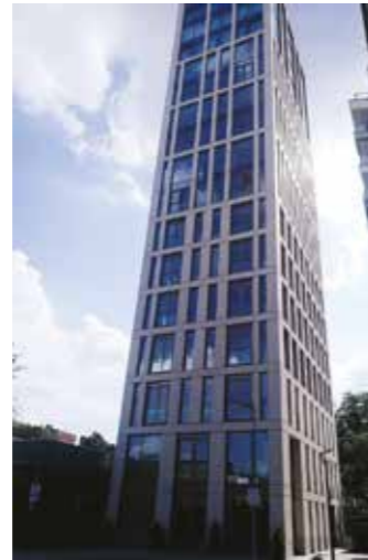
Gridded Facade with Solid and Transparent elements. Emphasis on the vertical. Top. Middle. Base.
