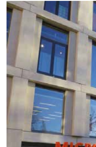
Secondary solid elements set back from the main grid to create relief
