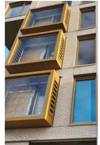
Option to pop out winter gardens at upper levels to add additional animation to the facade
