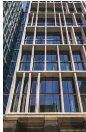
Introduction of secondary vertical elements (fins) to allow for playful articulation of the facade
