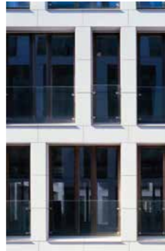
White, light coloured stone as principal material with tinted glass to create a strong contrast
